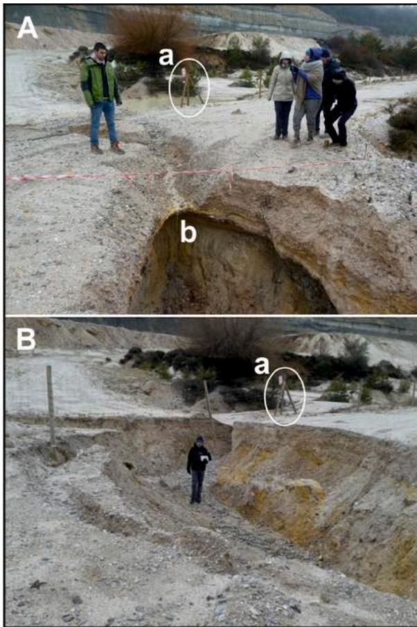
**Fig. 4.** Gully erosion cutting one of the roads in the Nuria mine. (A) knickpoint (b) migrating upstream (January 2016) and (B) erosion bisecting the road (February 2017). (a) the position of a wooden pole is used as reference. Modified from Hancock et al. (2020).
