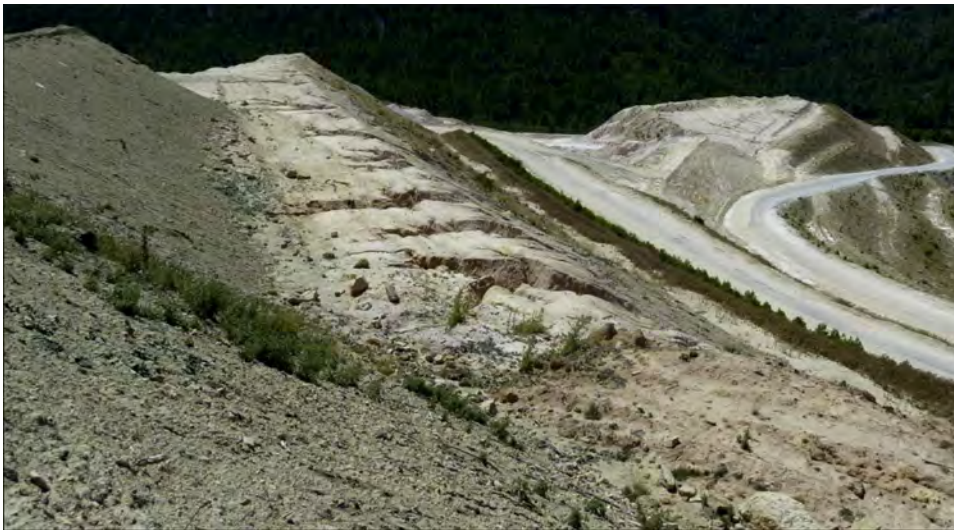
Fig. 17. Inversion of a berm slope by sediment accumulation at the toe of the upper outslope, leading to gullying downstream.
