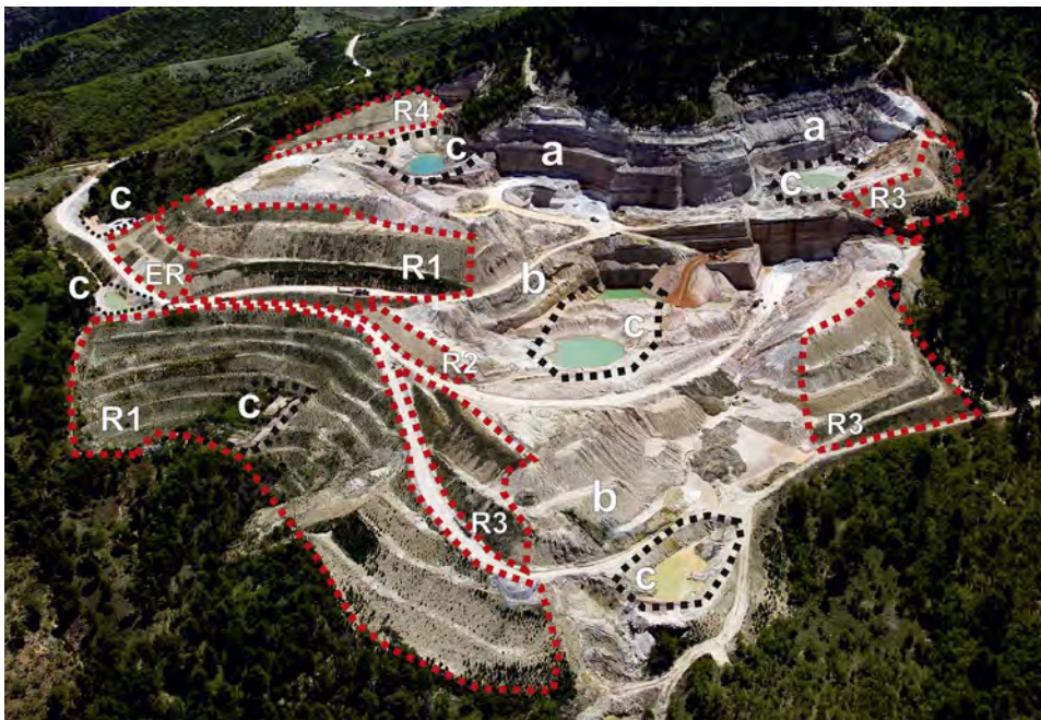
Fig. 4. Oblique aerial view of the El Machorro mine in 2014. Photo by Paisajes Españoles (2014). a, open pit; b, un-reclaimed waste dumps; c, ponds; R1, terraces covered with carbonate colluvium; R2, smoothed sloping terraces covered with carbonate colluvium; R3, terraces covered both with carbonate colluvium and soils; R4, geomorphic reclamation using GeoFluv-Natural Regrade (site of this study); ER = experimental mining reclamation waste dump.
