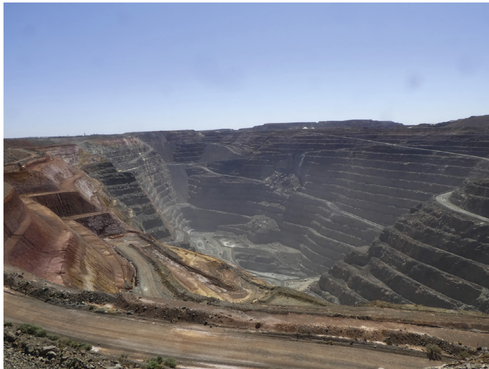
Fig. 8 The “Super Pit,” one of the Australia’s largest open pit mines, is located in Western Australia. The pit is oblong in plan and is ~3.5 km long, 1.5 km wide and over 500 m deep (Mossa and James, 2013). Photo: J.F. Martín Duque, September 2019.
