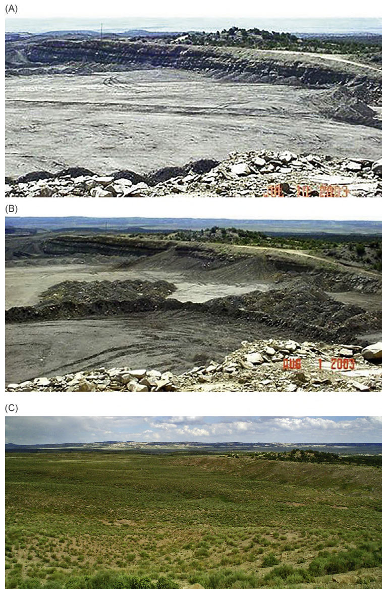
Fig. 10 Geomorphic restoration at La Plata mine, New Mexico (USA). (A) July 2003: prior to geomorphic restoration; (B) August 2003: beginning of placement of leftover earth material in accordance with the restoration design; (C) October 2010: reconstructed landscape five years after completion of grading, topsoil placement, and seeding. The distance across the pit in (a) is ~ 5 km. View is to the southwest; drainage is from right to left. Photo credits: Nicholas Bugosh.
