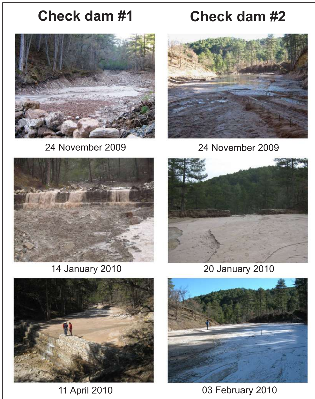
Figure 9. Check dam storage areas before and after the 10 December 2009–18 January 2010 period. Top: CD#1 under construction (3 m high) and CD#2 partially cleaned; middle: check dam storage areas completely filled by sediment; bottom: 4.5 m high CD#1 and CD#2 some months after the studied period, their storage areas were completely filled by sediment. [Colour figure can be viewed at wileyonlinelibrary.com ]
