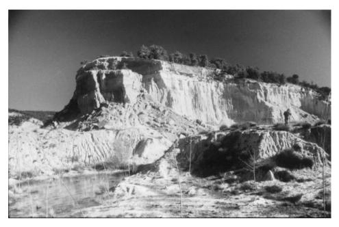
Fig. 2. General view of the west sector of the quarry prior to the rehabilitation: dispersed spoils banks affected by erosion processes, falling of blocks from the abandoned quarry face and significant impact on the ecology and landscape.
