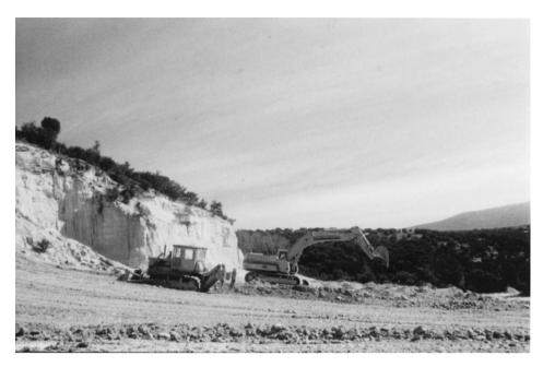
Fig. 9. The project was performed between January and February 1995. The picture shows the works relating to reconstruction of the glacis type morphology, and extending of the colluvial material on the final surface. Since the use of heavy machinery led to compactation of the terrain, decompactation work was subsequently carried out using the traditional farming techniques of the region (ripping, ploughing).
