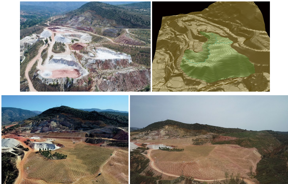
Figure 6 Western mine site of TECMINE. Upper left, aerial view pre-rehabilitation (July 2018, photo by Paisajes Españoles SA); upper right, 3D view of the GR design; lower left and right, aerial views after geomorphic regrading, colluvium spreading, seeding and planting (photos by Vaersa)
