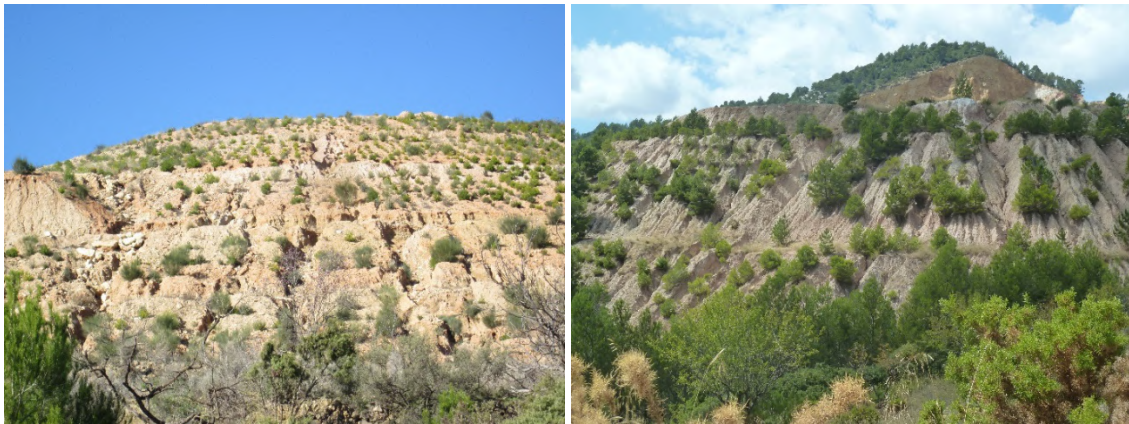
Figure 4 Conventional waste dump mine rehabilitation in the Valencian Iberian Range; terraced landforms with Mediterranean pine, showing widespread gullying (photos by José F Martín)
