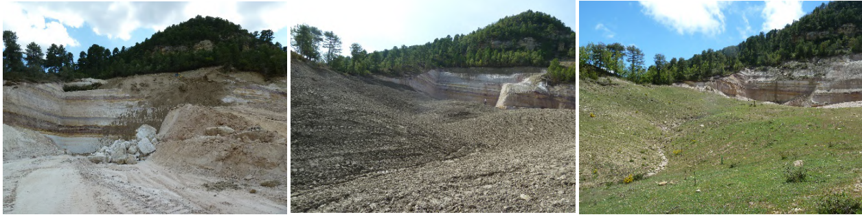
Figure 1 Geomorphic rehabilitation of a sector of El Machorro kaolin mine (Poveda de La Sierra, Guadalajara, Spain). Left, before rehabilitation (August 2012); centre, after landform regrading and soil replacement (October 2012); right, first stages of vegetation re-establishment (May 2014). Photos by José F. Martín
